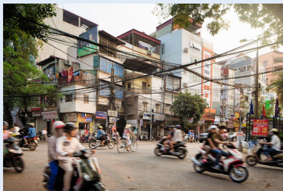
Figure 1.5: Power lines supply electricity to buildings in Hanoi, Vietnam.
