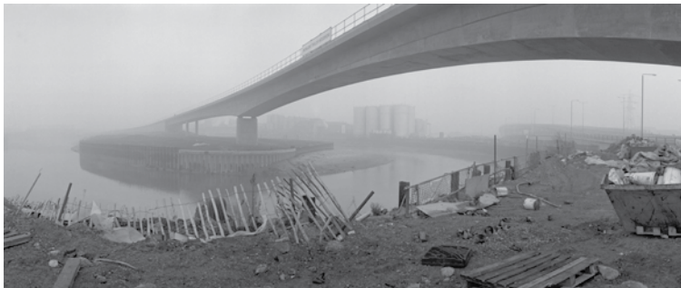
Docklands Light Railway crosses the River Lea in East London, site of the 2012 Olympics Park; 1992
